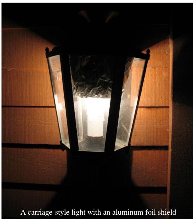
A carriage-style light with an aluminum foil shield
